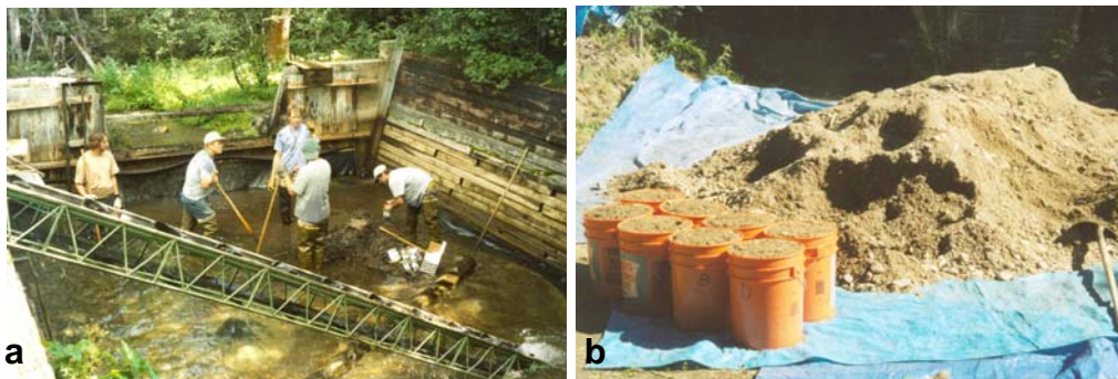
Figures 5 a and b: Excavation of the lined debris basin (a). Excavated debris pile on a tarp with samples being collected (b)
