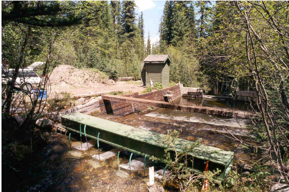
Figure 2: Four bedload traps installed in front of a footbridge just upstream from the East St. Louis Creek debris basin. Note the gauging hut and the weir in the background.
