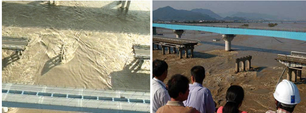
Figure 9. Gupo bridge failure after Typhoon Maemi [Yonhap]
