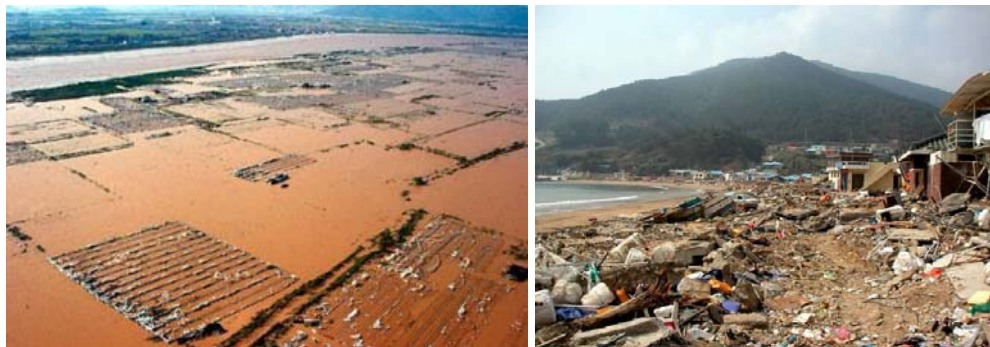
Figure 7. Flood damages of Pusan of left, [AP] and Wah Yeon Beach on Geoje Island of right, [photo by Paul J. Riley]
