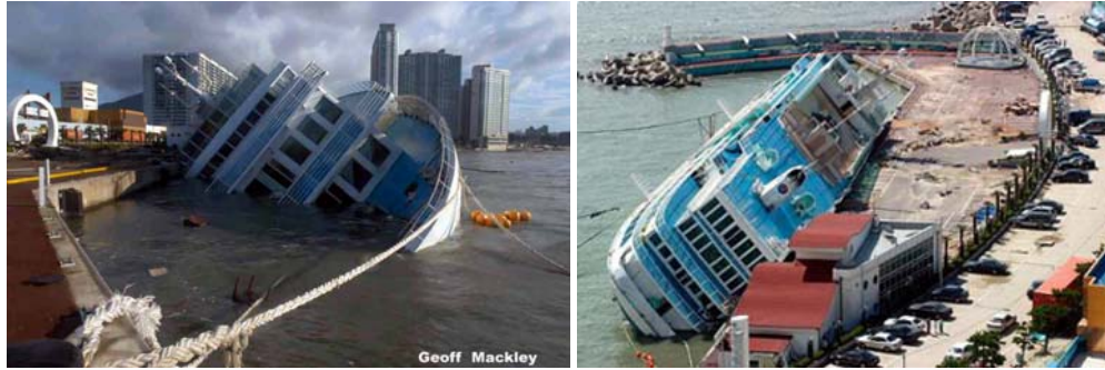
Figure 8. Damages of ferry-shaped hotel after Typhoon Maemi hit Pusan Port [AP]
