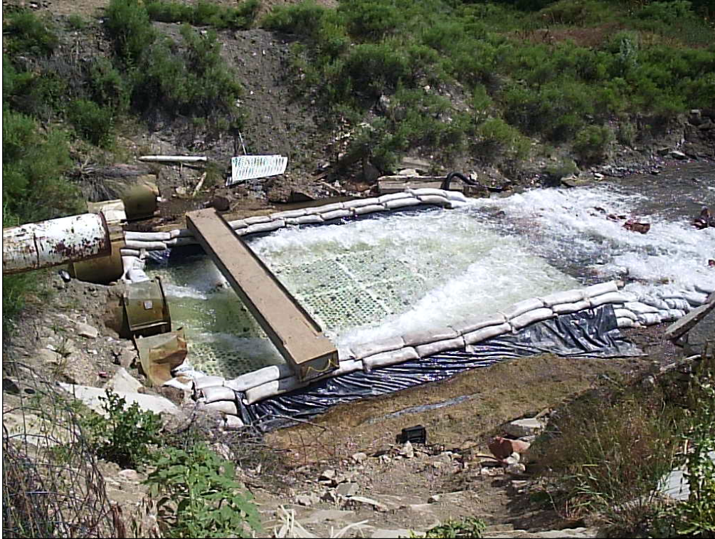
Figure 1. Full-scale culvert outfall testing at CSU
