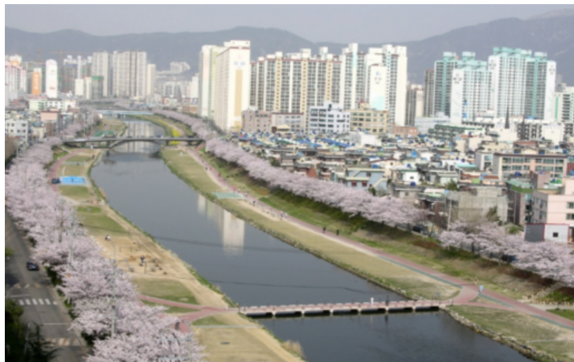
Fig. 2. A view on Sebyeong bridge site
