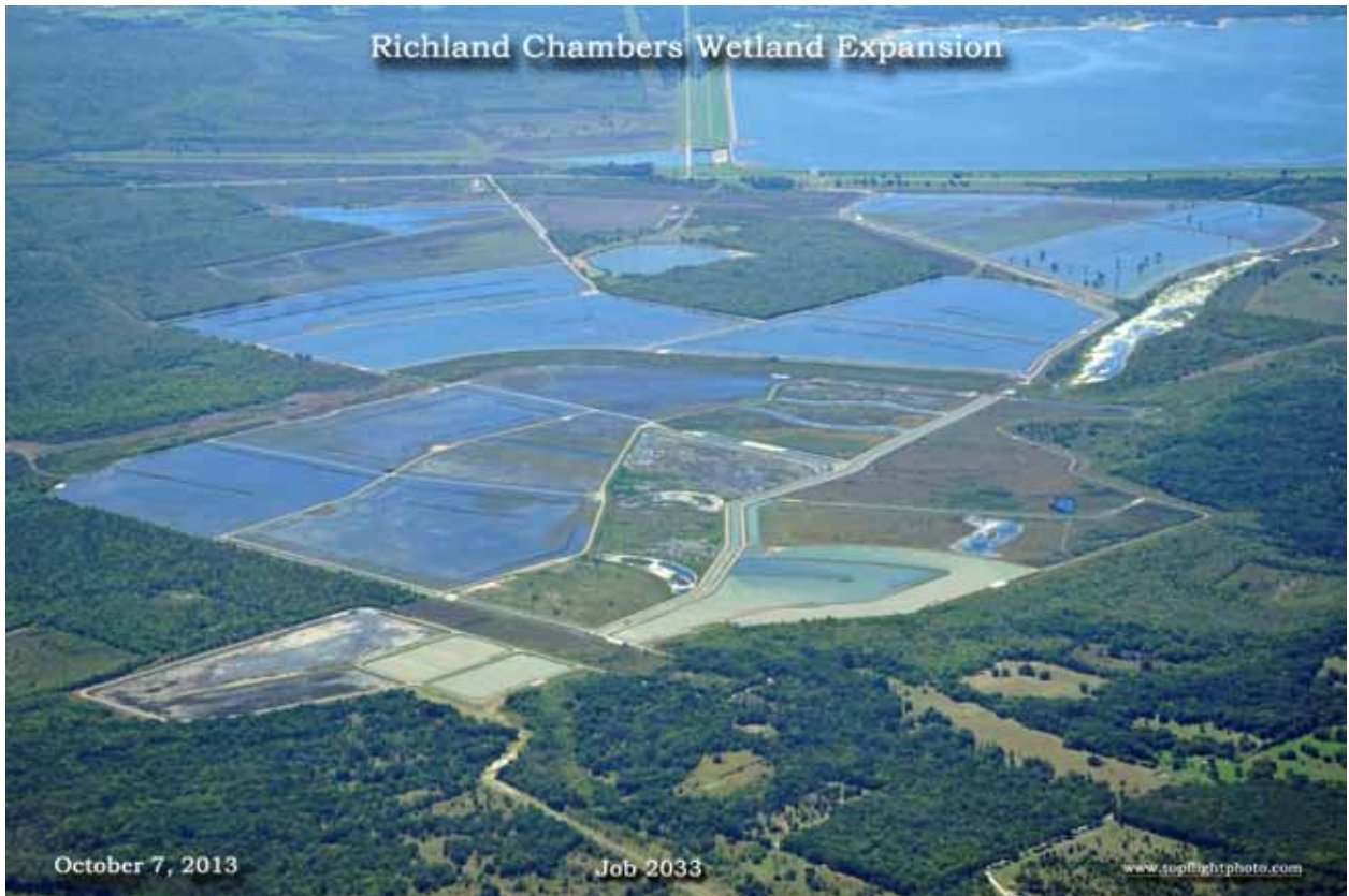
Figure 10. Completed and operational Richland Chambers Wetlands Facility.
