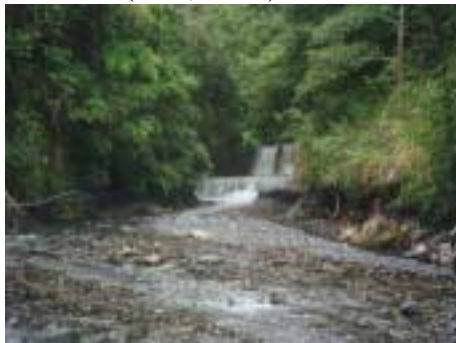
Photo 11. Dam No.3 before construction (Oct., 1997)
