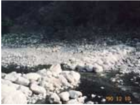
Photo 1. Rock weir of partial width
