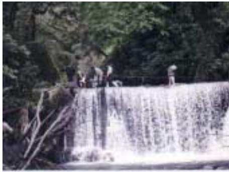
Photo 9. Dam No.4 in construction (April, 1999)
