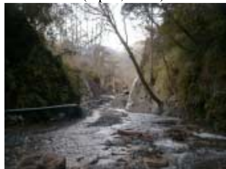
Photo 16. Dam No.1 recent condition (Dec., 2001)
